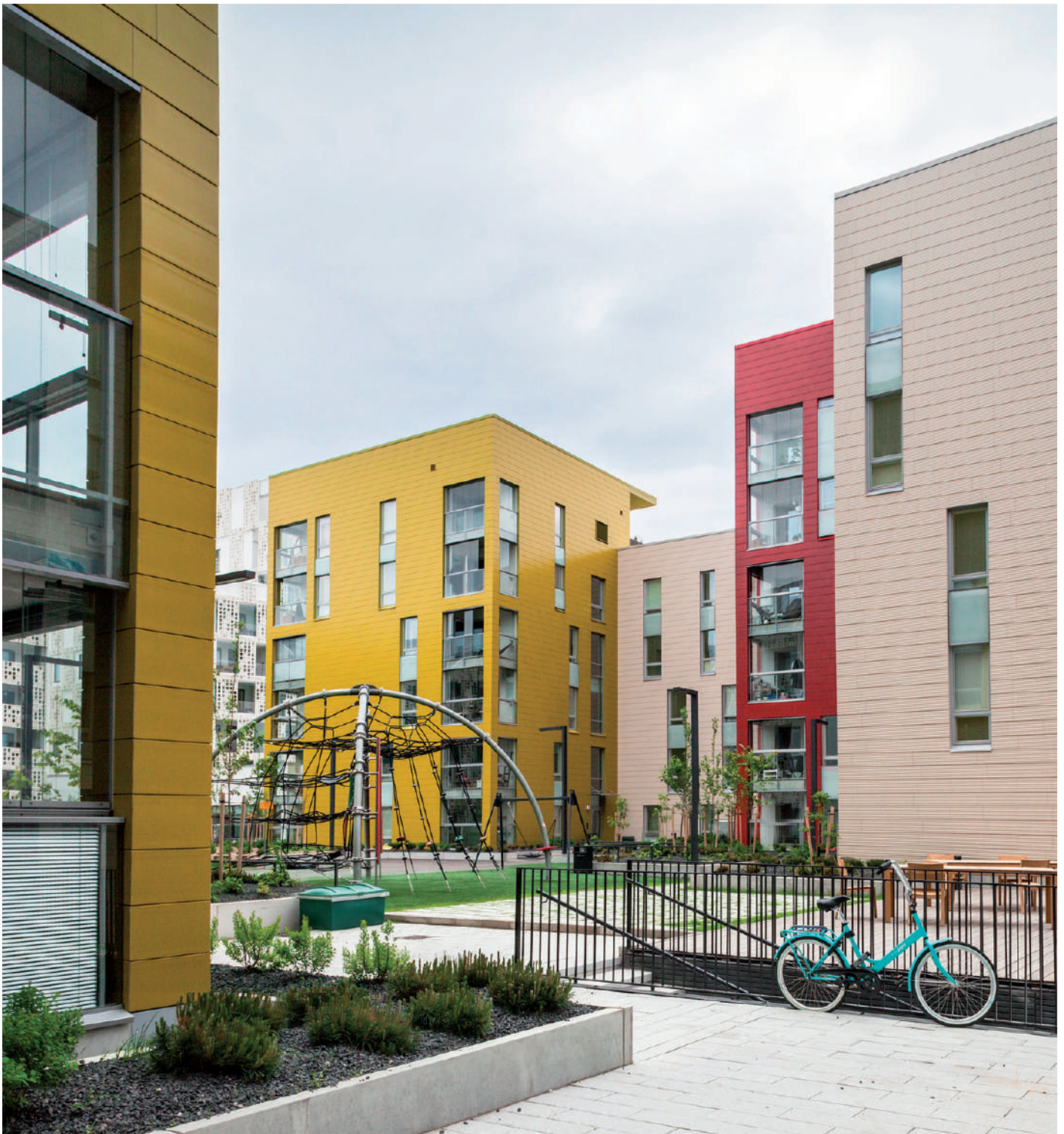
tempio®[projects] Saukonkanava, Helsinki, Finland.
